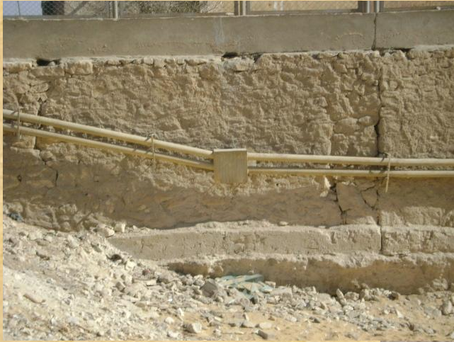
BEFORE CLEAN UP
