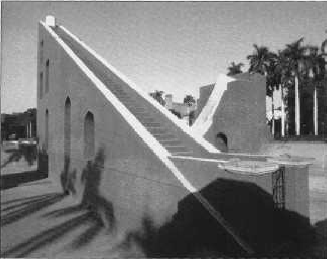
[29. The Samrat Yantra, or giant sundial (a masonry gnomon) in the observatory at Jaipur. It is still an accurate time-keeper for the city, which is regulated according to solar time.]
